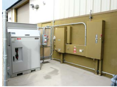
Solar System capable of producing 8,000 kWh monthly
