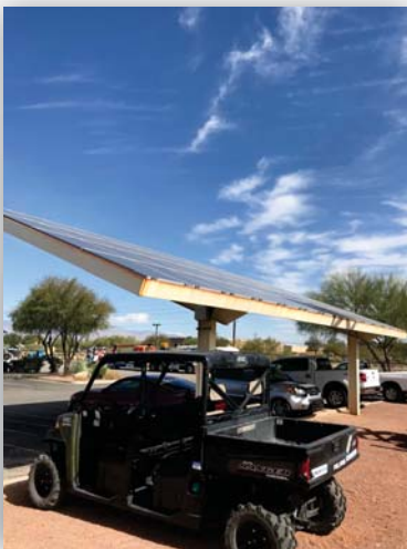
Covered Employee Parking
